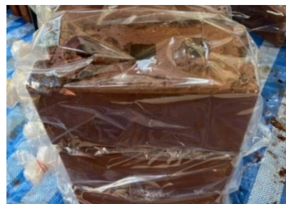
Fig. 3 Curing interlocking block with plastic bags
